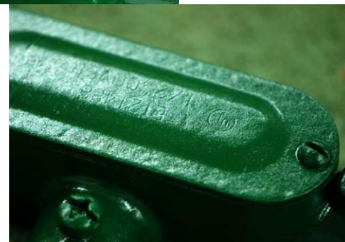
Conduit after dobbling.
