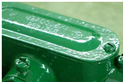
Conduit painted, but before dobbling.
