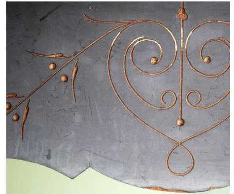
Detail prior to restoration
