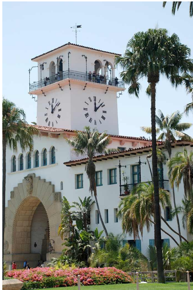
Santa Barbara Courthouse Tower Clock
